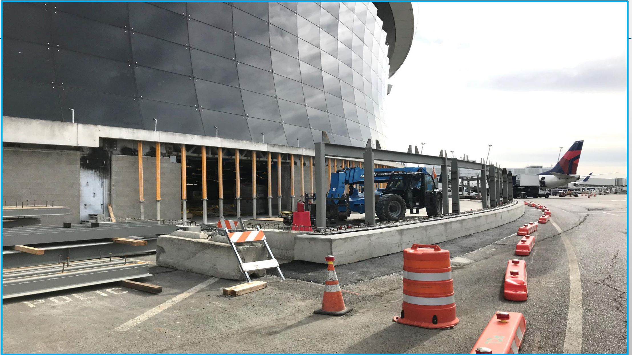
CTE Bump Out – Steel Installation
